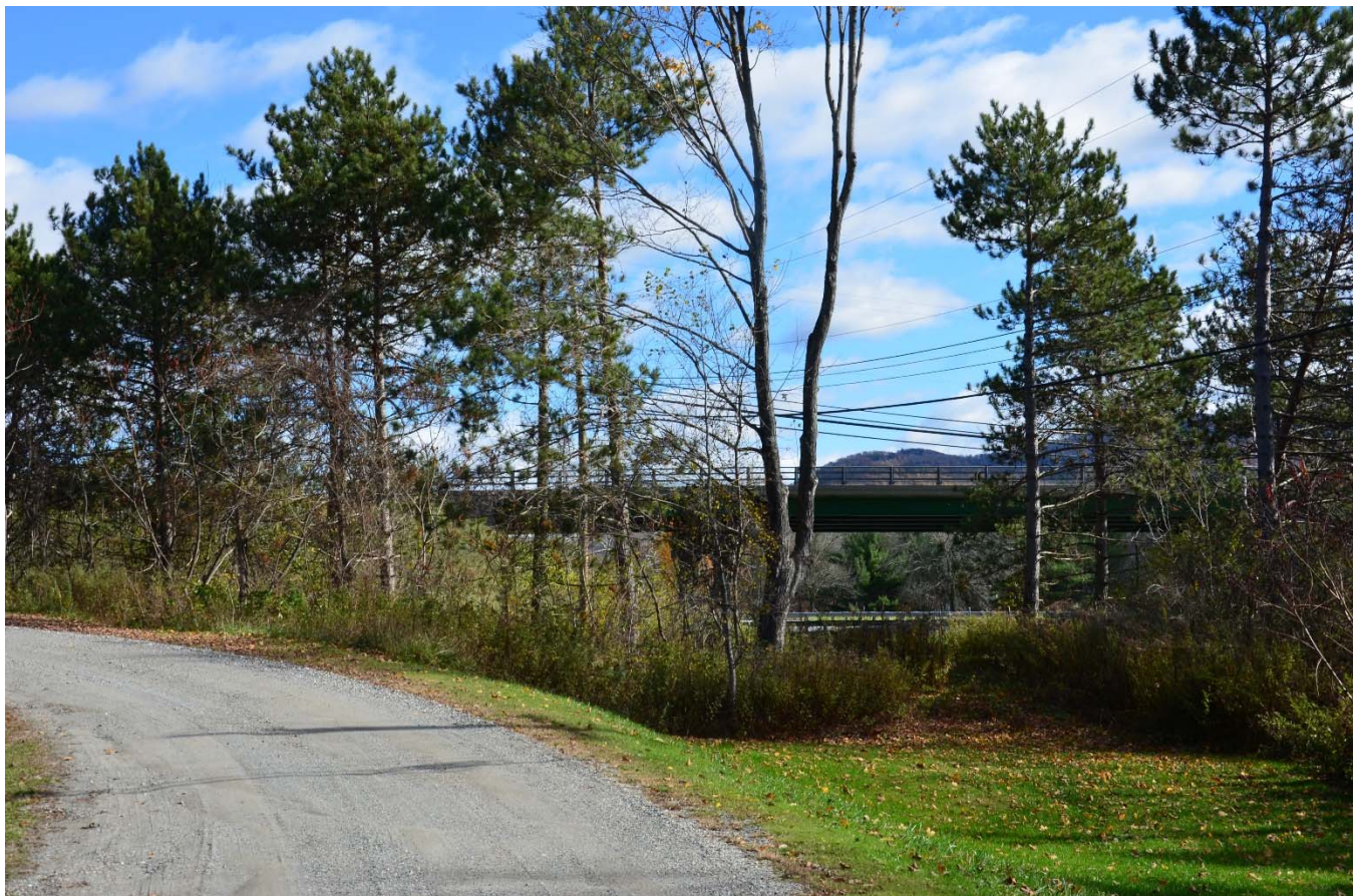
Viewpoint 31: View looking east from Higgins Road toward the East Hubbardton Road overpass at Exit 5, US Route 4.
