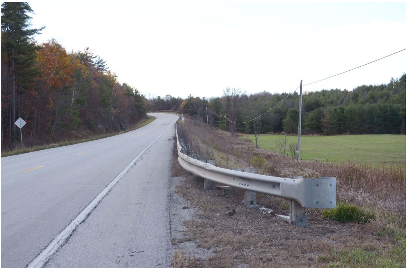
Viewpoint 22: View looking south along the highway embankment near MP 106.9. The line will run along the base of the slope and then merge back to the edge of the shoulder along the edge of the background vegetation.
