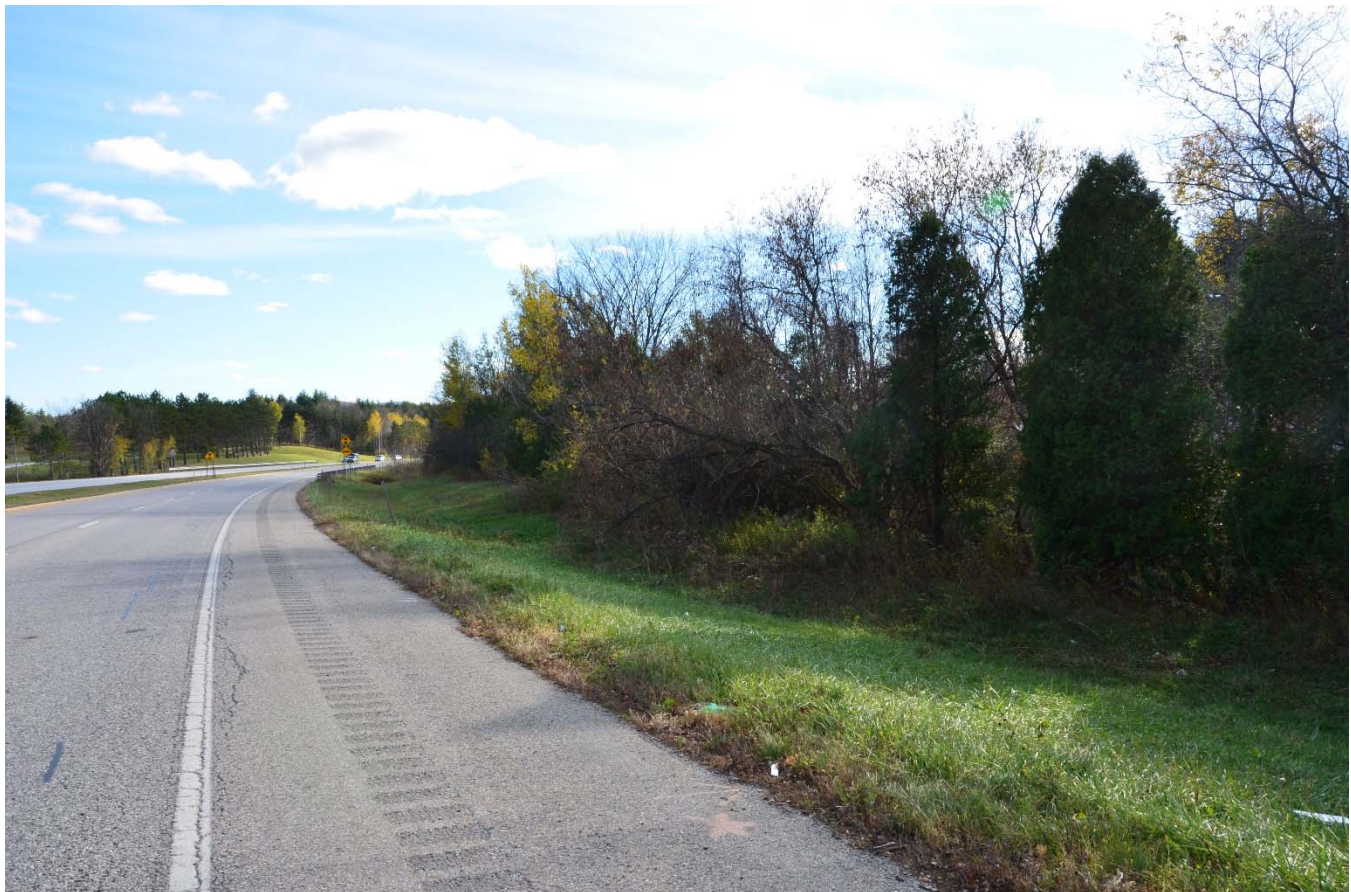
Viewpoint 47: View looking at a thin buffer of vegetation within and adjacent to the HDD staging area south of the Cold River crossing along US Route 7. * Wide Angle Zoom
