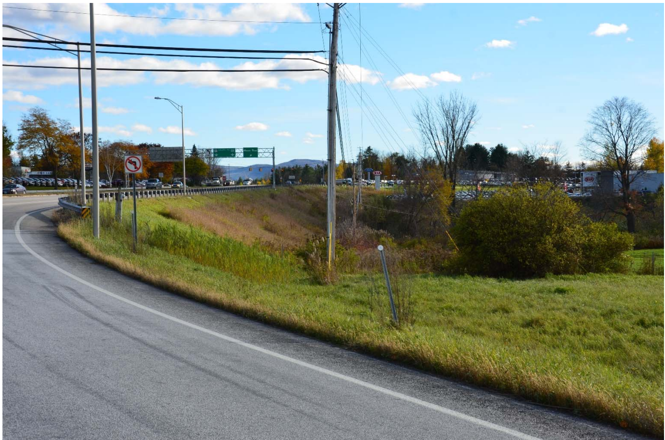
Viewpoint 45: View looking at the HDD staging area at US Route 7. The existing overhead utilities will need to be relocated.
