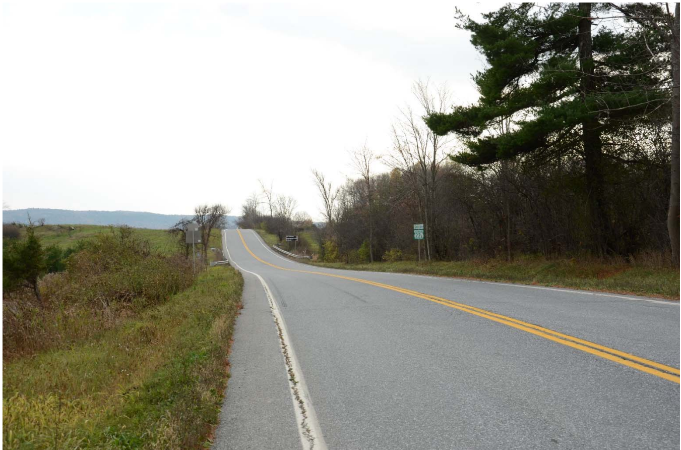
Viewpoint 13: View looking south along the eastern shoulder of Vermont Route 22A at the intersection with Hulett Hill Road. The line will be installed outside of the eastern shoulder of the road.
