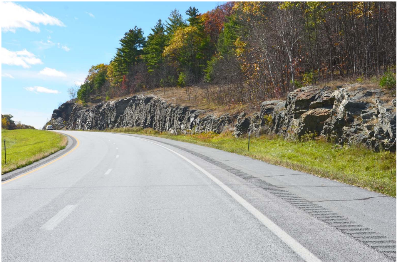
Viewpoint 36: View looking west along the westbound lanes of US Route 4 at typical section of the Project where the line will be installed between the paved shoulder and an adjacent rock cut.
