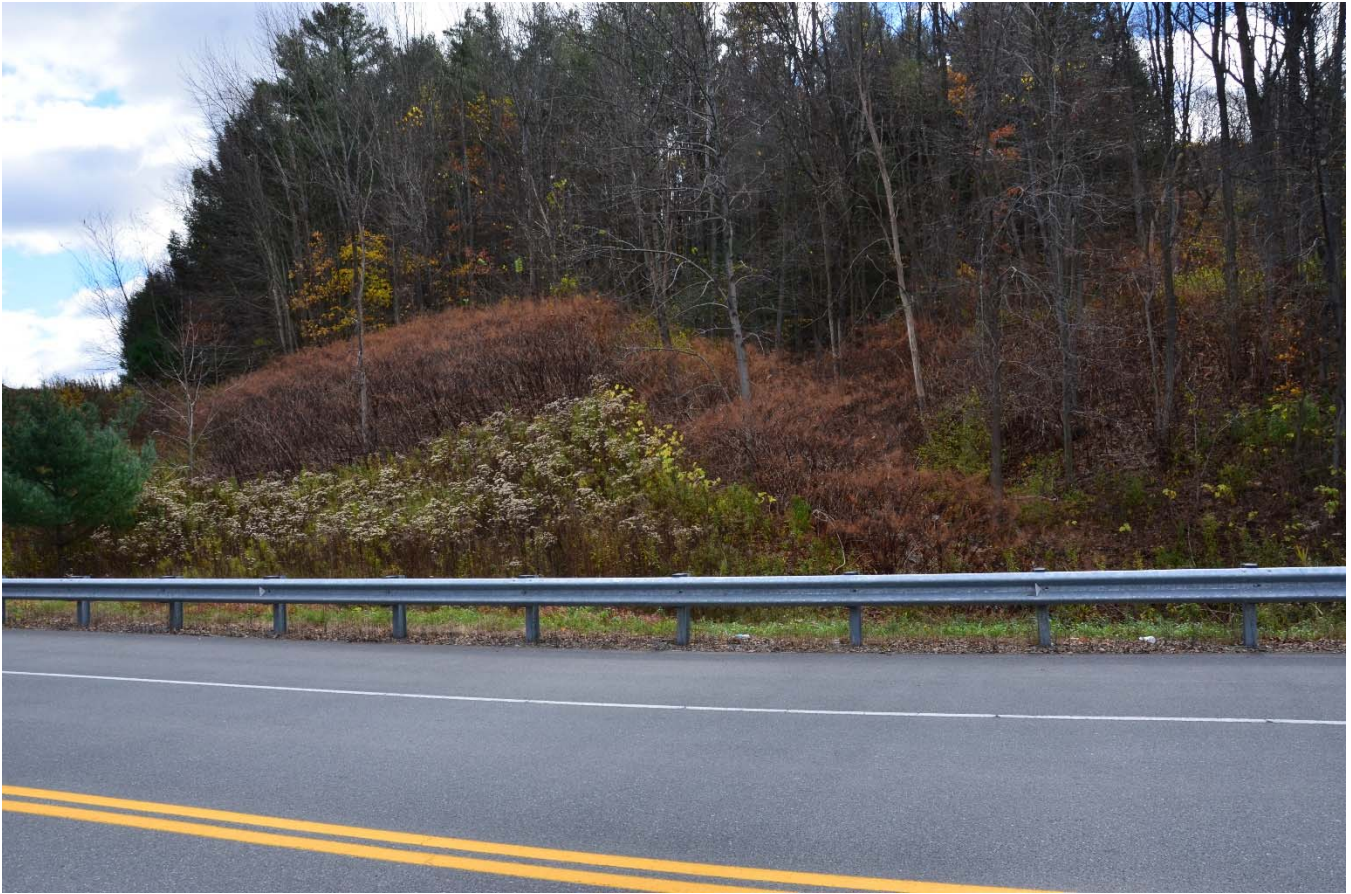
Viewpoint 24: View looking southeast from Route 4A after the line has crossed beneath US Route 4 and will continue east along the southern edge of the eastbound lanes.
