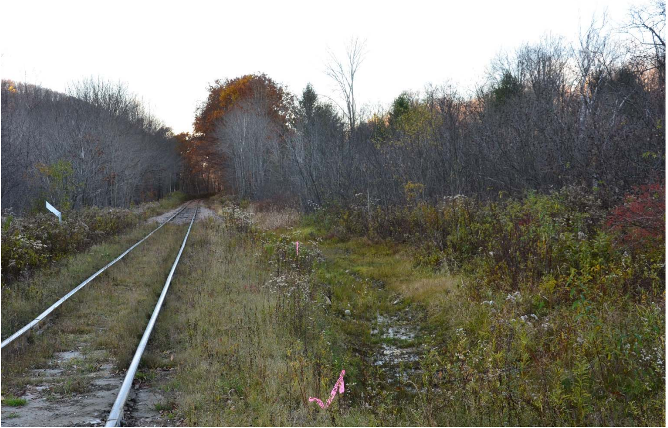
Viewpoint 67: View looking north at HDD staging area in foreground. The woods in the mid and background along the north (right) side of the tracks will be cleared 40 feet back from the edge of the closest rail.
