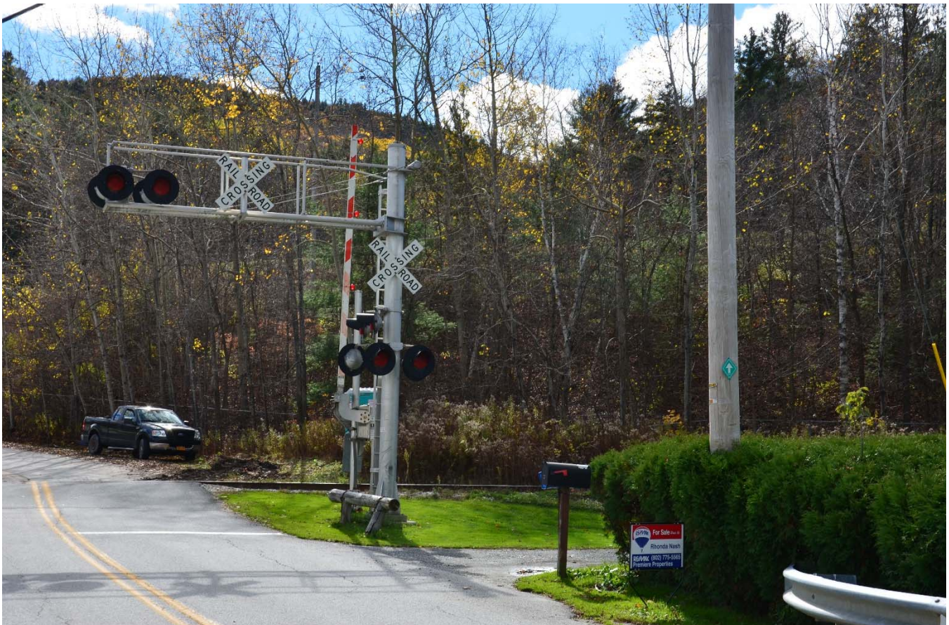
Viewpoint 25: View looking south at vegetation on the US Route 4 embankment that will be cleared for a HDD staging area. Clearing of this vegetation will remove the buffer between Route 4 and Whipple Hollow Road and the surrounding properties.
