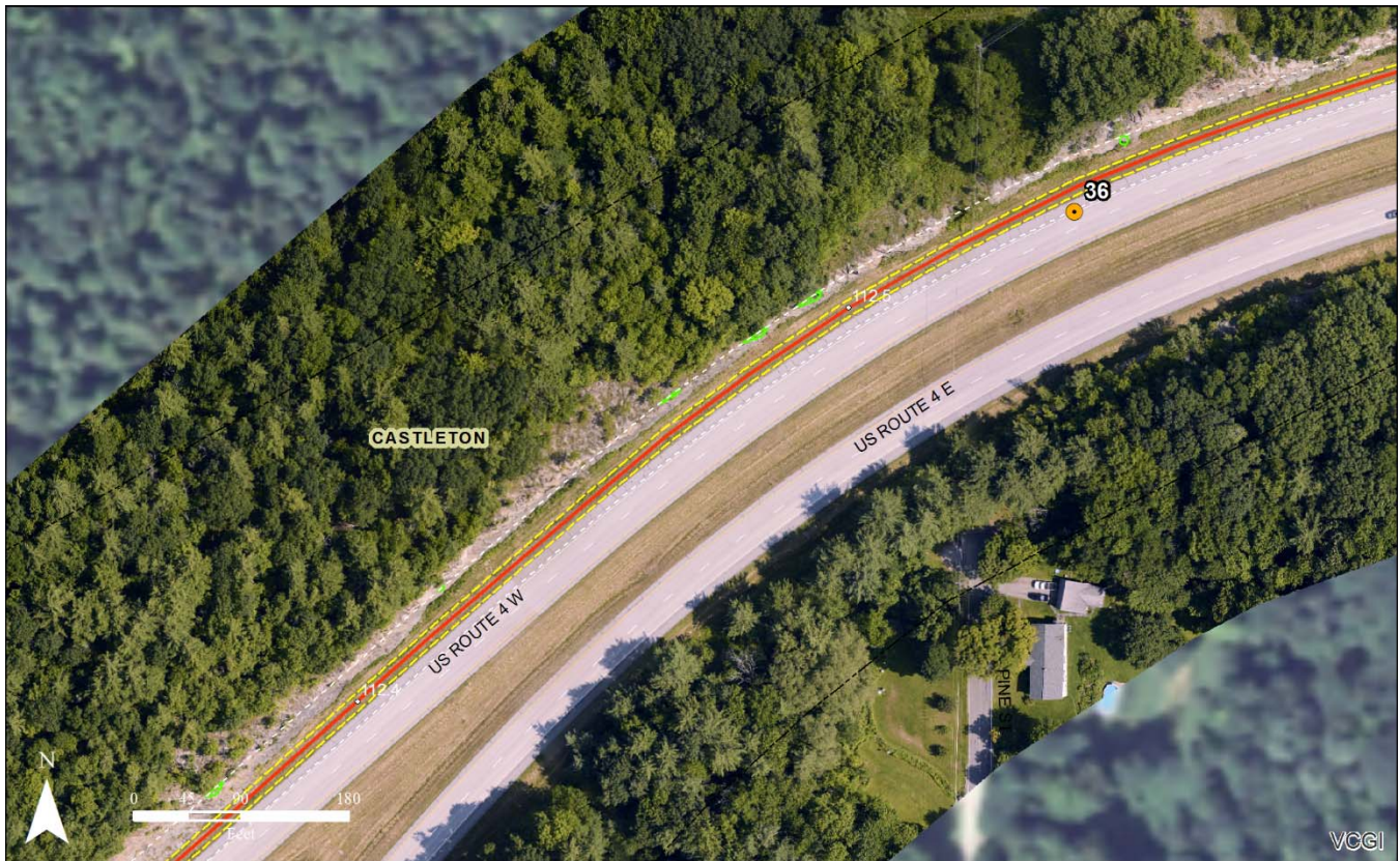
Assessment Map 18: A typical section of the Project along US Route 4 where the line will be installed between the edge of the paved shoulder and a rock cut.
