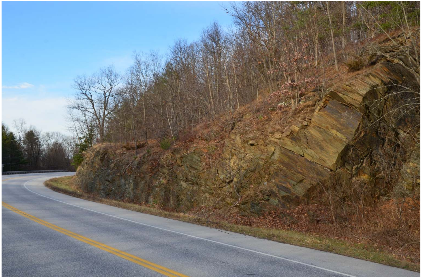
Viewpoint 110: View looking north along Vermont Route 22A. Construction of the line at this location may require the existing face of the ledge to be removed and widen the clear zone along the highway where the cable will be installed.
