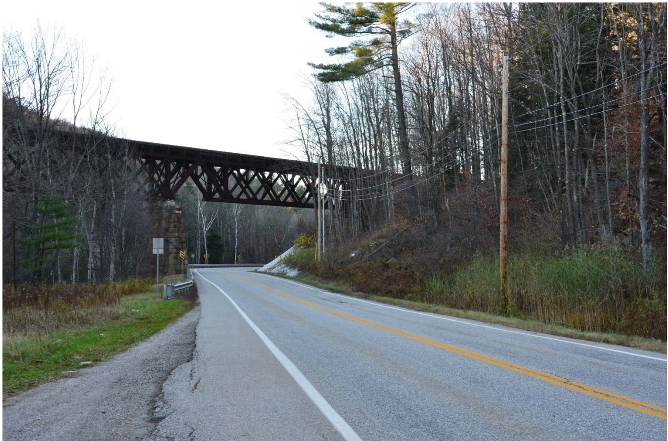
Viewpoint 69: A 50-foot wide corridor will be cut alongside the railroad where the line descends the slope to meet with Vermont Route 103 and clearing for a HDD staging area is proposed at this location.
