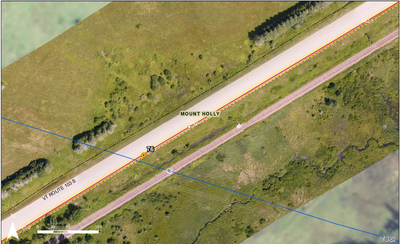
Assessment Map 44: Another example further east along Vermont Route 103 in Mount Holly, illustrating the wide open areas along the road, which will allow the Project to be installed with little visual change after construction is completed.
